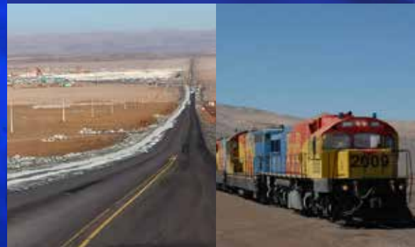
Quality Road & Rail Infrastructure
